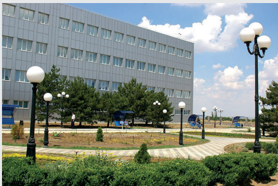
A regional dispatch center building, Simferopol, June 15, 2007. Photo from Ukraerorukh official website
