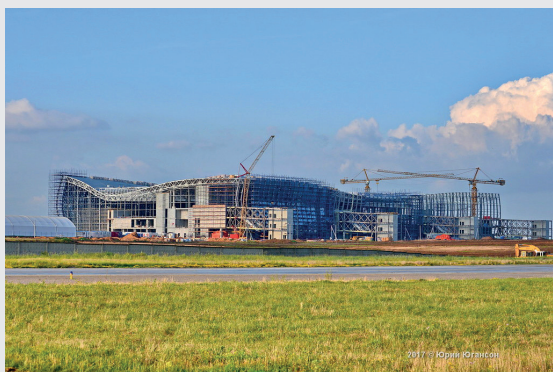
New terminal construction, Simferopol airport, July 2017. Photo from BlackSeaNews archive
