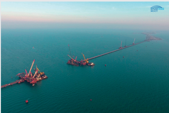
Construction site of the navigable bridge span, November 2016. Photo from www.most.life
